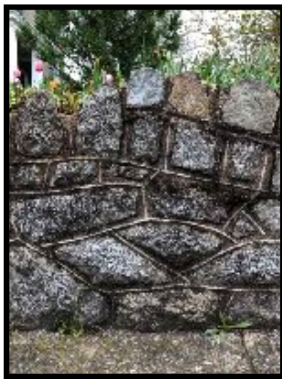
An example of “Rock Creek Granite” and beaded mortar
