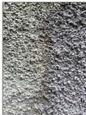
A seamless pebble dash repair just waiting for paint. (Photograph by MaryAnn Nash.)
