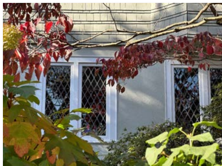
Windows designed with diamond muntins. Photograph courtesy of MaryAnn Nash.
