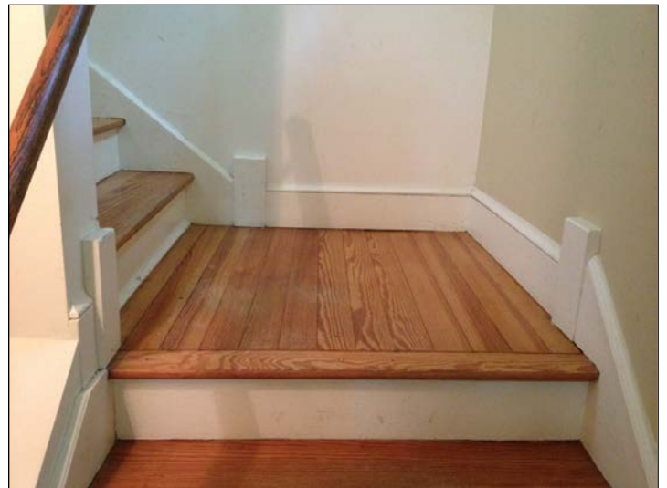
The stairs in the Hanson house, a Sears "Walton." The plinth blocks where the pieces of stair molding meet are specific to Sears kit houses. They were designed to help homeowners inexperienced in carpentry handle complex baseboard angles if they were building the house themselves. (Photo by Catarina Bannier)
