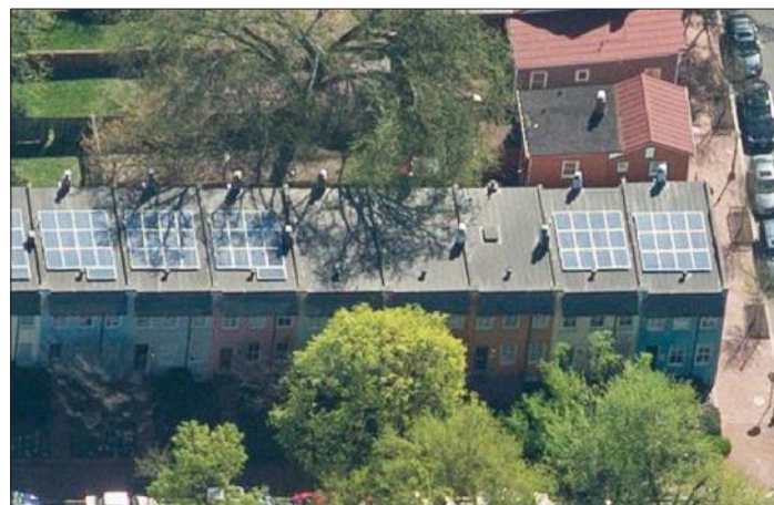
PANELS INSTALLED ON THE FLAT ROOFS OF THIS ROW ARE IMPERCEPTIBLE FROM THE STREET, HIDDEN BY PARAPETS AND PENT ROOFS.
