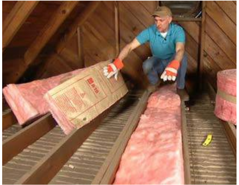
BATT INSULATION BETWEEN THE CEILING JOISTS
