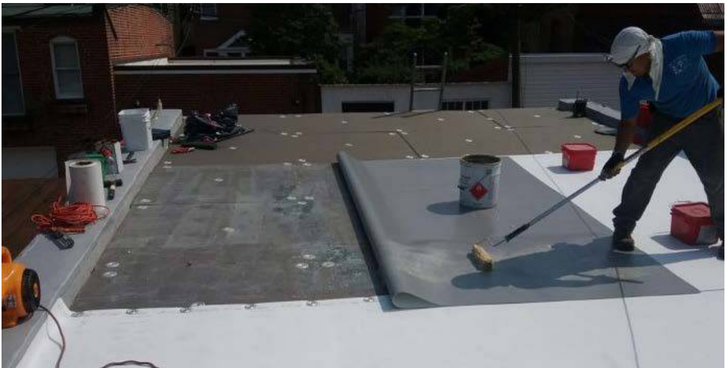
ROOF MEMBRANE REPLACEMENT
