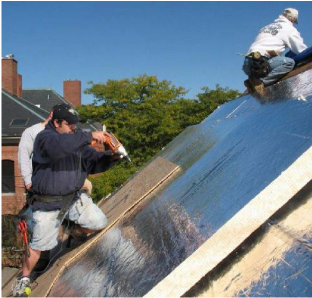
RIGID INSULATION ON A SLOPED ROOF
